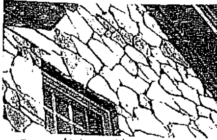
Fig. 3. Flint walling or Flint Rubble masonry
