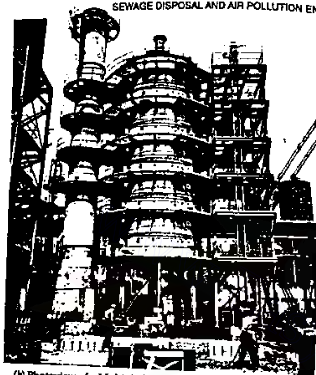
(b) Photoview of a Multiple-hearth Incinerator Installation
