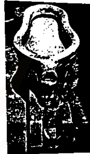
Fig. 12.6. Sulabh pan mounted on sulabh seal.
