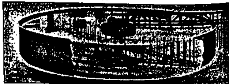
(c) Photoview of a gravity sludge thickener
